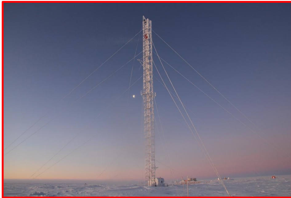
45m tower, 6 levels of measurements
