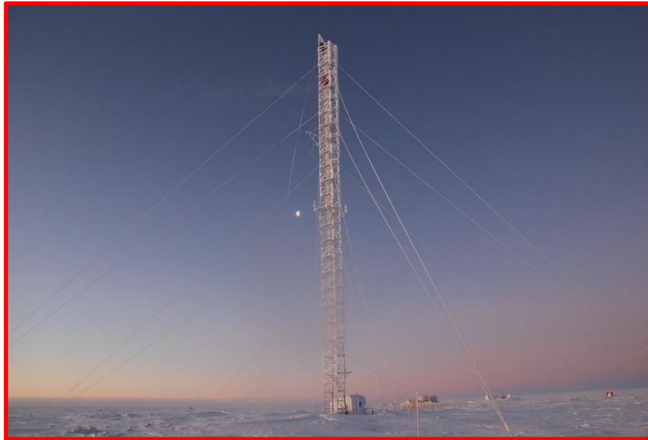
45m tower, 6 levels of measurements
